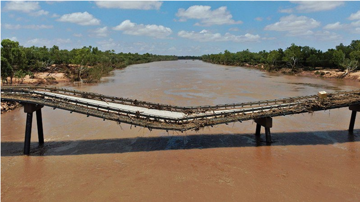
Image: New Fitzroy River Bridge Project, Western Australia (Source: Main Roads WA, 2023)
