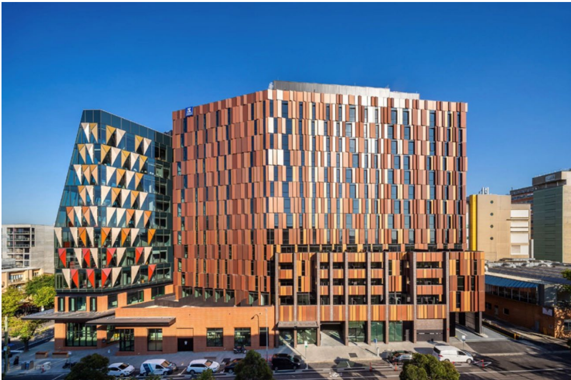
Melbourne Connect building (ANZSOG HQ) Photography: Peter Casamento
